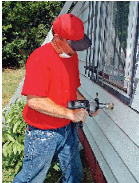
Right: Older homes can be retrofitted with blown-in insulation. Below: Volunteers caulk and paint a home for Habitat for Humanity. Caulking is a simple way to prevent air leaks.
